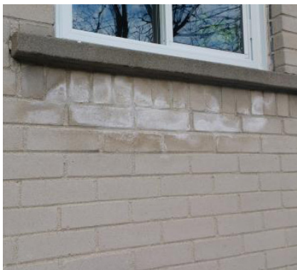
Some more examples of efflorescence on coloured concrete paving and brick.
